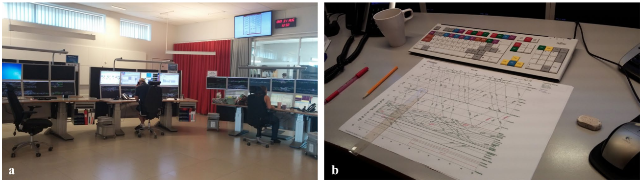
Fig. 2 a To the left, a control room and three workstations for traffic control. b To the right, the main artefacts used for controlling the traffic (the traffic control system, the time–distance graph, and the telephone)
